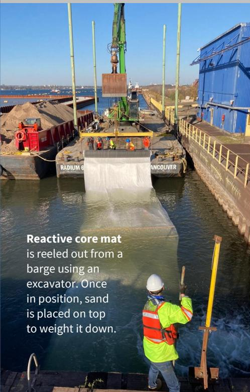
**Reactive core mat** is reeled out from a barge using an excavator. Once in position, sand is placed on top to weight it down.
